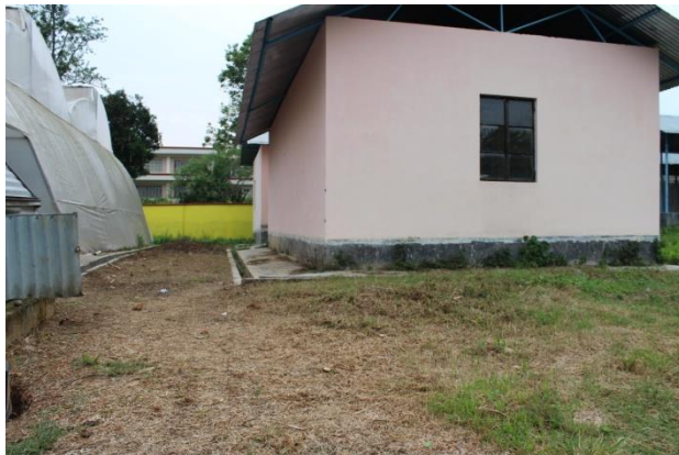
Cleaning of area behind PH structure
