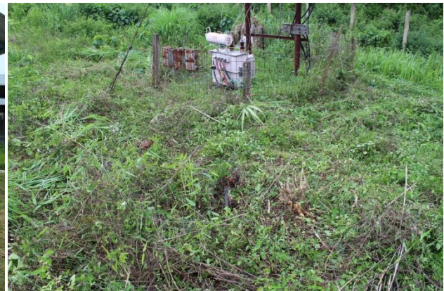
Jungle clearing near power station
