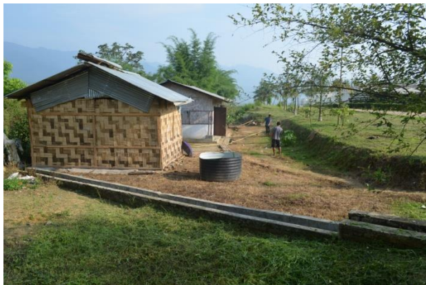
Cleaning of area behind mess hall
